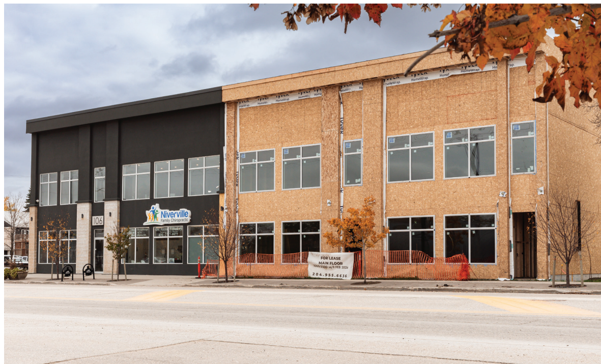
A large new addition is underway at 106 Main Street in Niverville.
