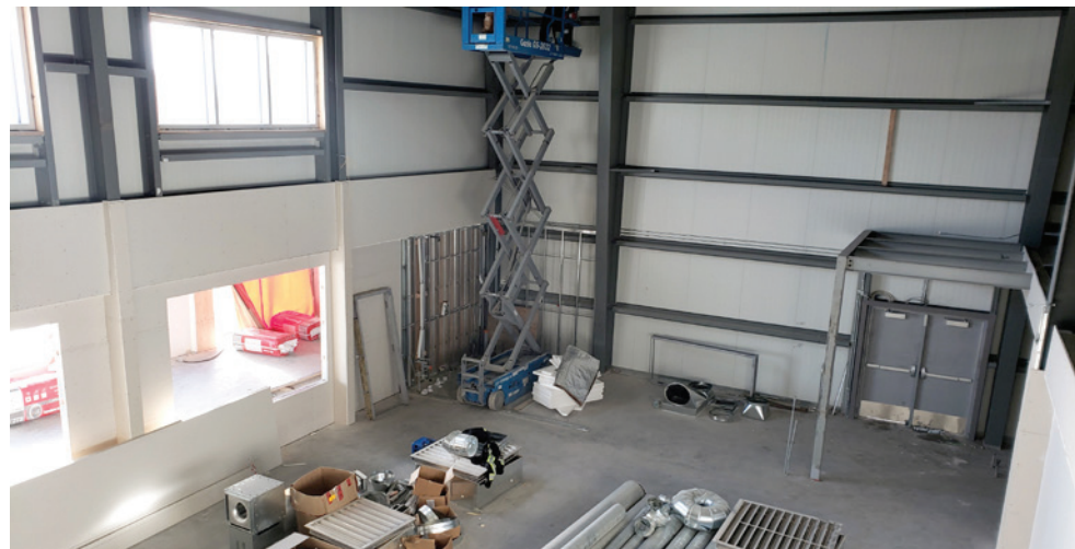
Drywall is being installed in the large foyer area inside the building's entrance. Once complete, this front area will include an indoor playground.
