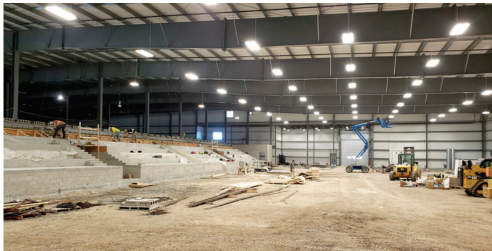
On the arena side of the building, seating has been installed. Concrete has yet to be poured over the ice surface.
