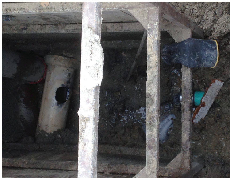
The point where a new connecting line, once installed, will feed into Main Street’s sewer main.
