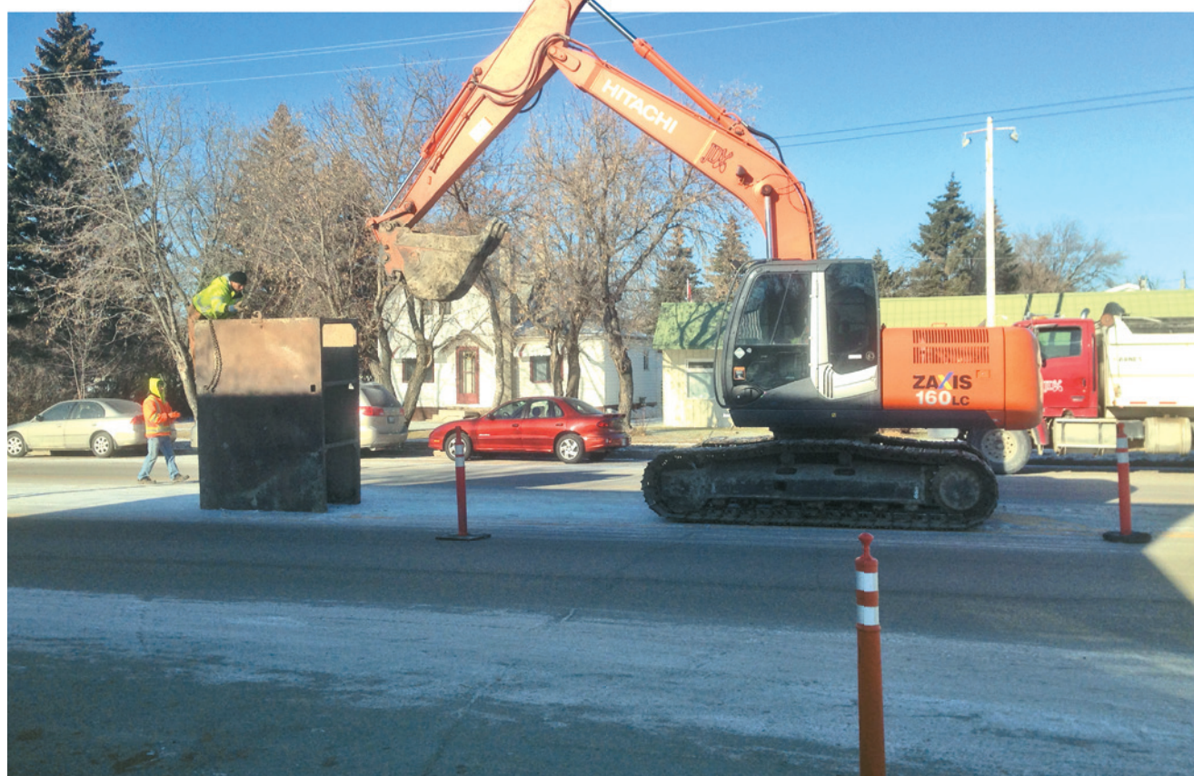
Excavation underway on Main Street to repair a sewer connecting line.
