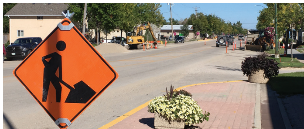
Installation of the new water line on Main Street Niverville.
