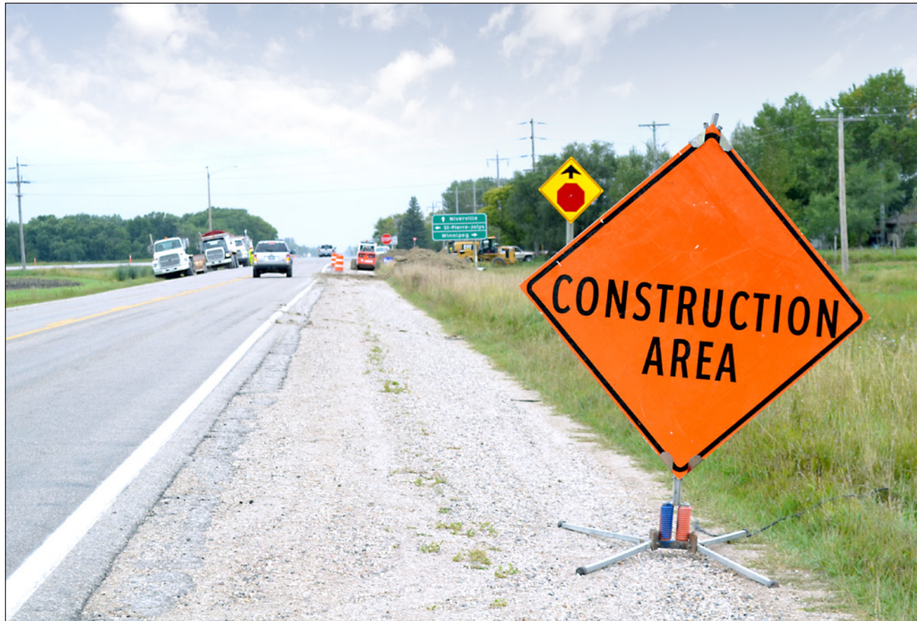
Construction crews begin installing signal bases.
