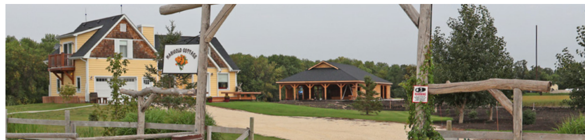
The new pavilion under construction at Whitetail Meadow.
