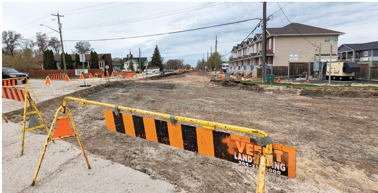
Major repair work is currently underway on Main Street in Île-des-Chênes.
