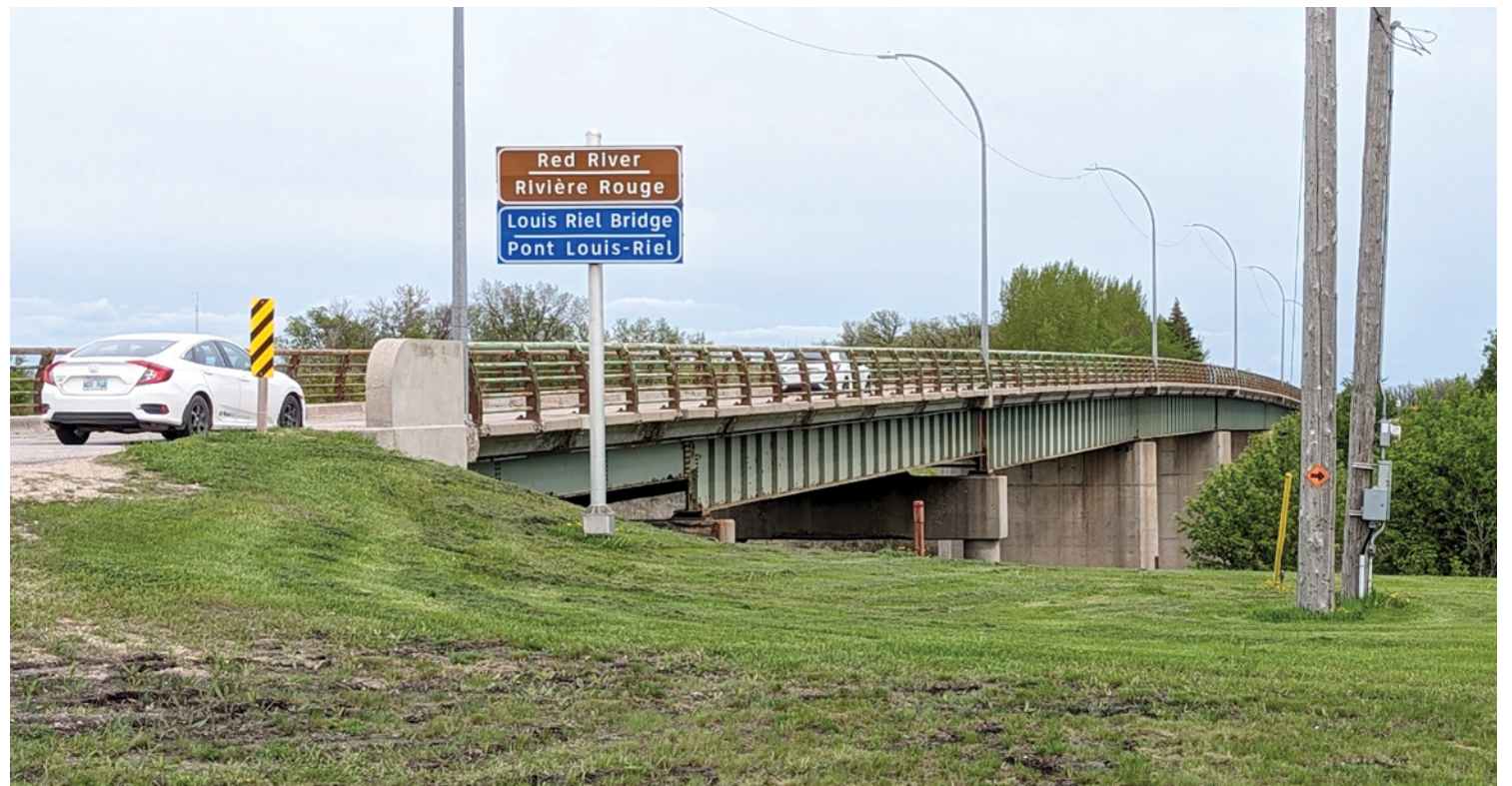
The Louis Riel Bridge in Ste. Agathe is about to get a major overhaul.
