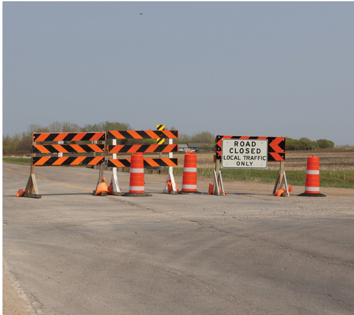
Since May, traffic has been rerouted around a burned-out bridge on Highway 311.
