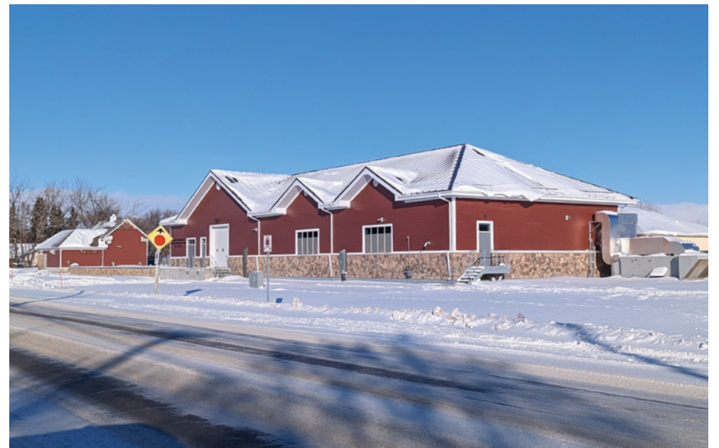
The water treatment plant in Niverville.
