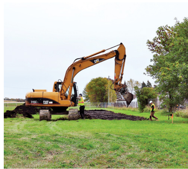
The excavation at 420 Main Street in St. Adolphe.
